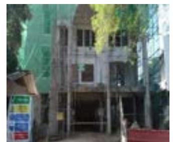
New office building underway.
